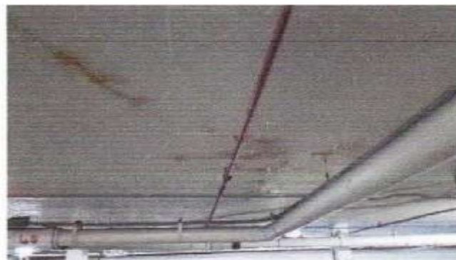
Previously installed and failed injection repairs
