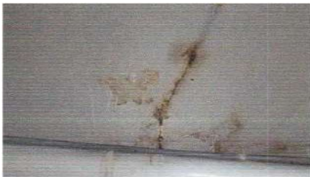
Previously installed and failed injection repairs
