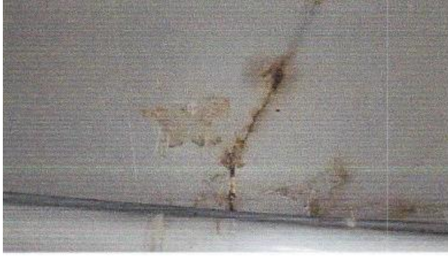
Previously installed and failed injection repairs
