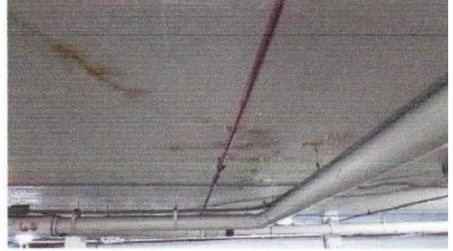
Previously installed and failed injection repairs
