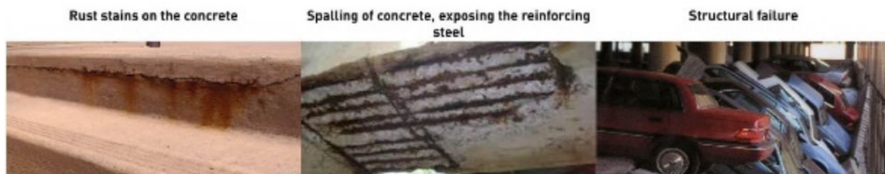
Stages of visible deterioration.
